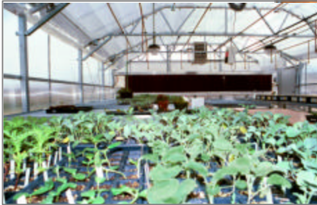
Power & Heat For Greenhouse
